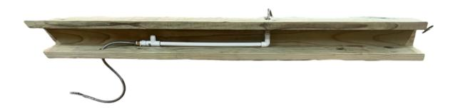
3. Apply PVC primer around the end of the pipe thats attached to the garden hose spigot, followed by PVC glue. Then insert the end of the pipe through the hole and into the PVC tee as far as it will go as shown below.
